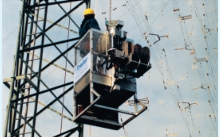
Powered end sections used as work baskets.
