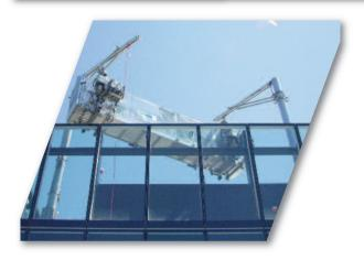
The Tracmod powered platform is fitted with the latest in Tirak powered hoisting systems, with all code-required safety feature fully intergrated.
