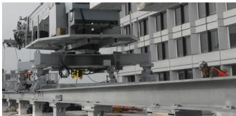
BMU's can be fixed stationary if the boom reach allows, if not a track on the roof is required for traversing the rooftop. The track will require a clear path of travel for the BMU free of obstacle's like air conditioning units or water tanks. BMUs are primarily run on a structurally anchored wide flange track near the edge of the building. Other options such as freely laid rail or concrete runways may be considered depending upon the application.
