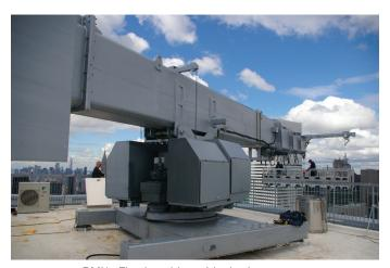
BMU - Fixed position with slewing turrent, telescopic boom retracted
