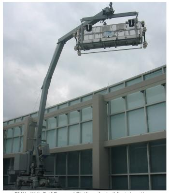
BMU - With Self-Powered Platform for buildings less than 490 feet
