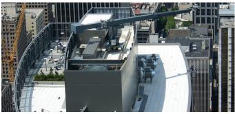
BMU - telescopic mast raised, telescopic boom deployed
