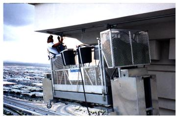
Example of Monorail used to suspend a TRACMOD Powered Platform – Caesar's Place, Las Vegas
